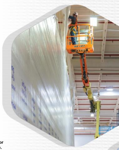
Hybrid Walls and Industrial Hybrid Walls are two types of hybrid dust walls that provide stability and resilience in high-traffic areas. The temporary walls help maintain a professional appearance during construction and protect inventory in the warehouse and retail settings. Hybrid Walls combine a C.O.R.E. Frameless Wall with TuffWrap's rigid TuffPanel® and with or without a pre-manufactured metal brace. Hybrid Walls are modular in design for clean, easy installation.
