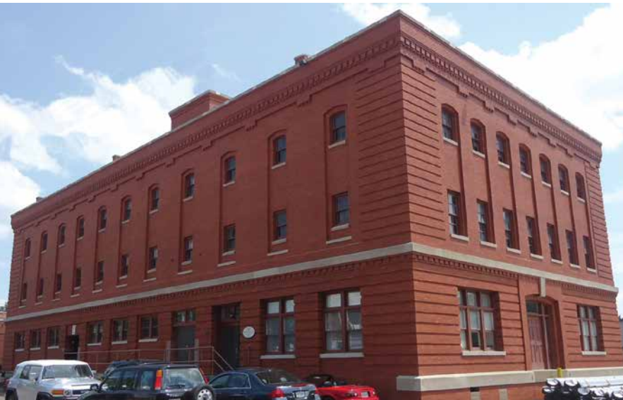
MFM Building Products Corp. Headquarters in Coshocton, Ohio.
