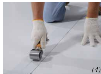
Peel & Seal® PowerBond™ White 250 installs in just four easy steps. (1) Wipe surface clean with acetone. (2) Peel back release liner. (3) Apply to seam of panels. (4) Roll seam for a tight and secure seal.
