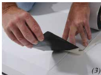
Peel & Seal® PowerBond™ White 250 installs in just four easy steps. (1) Wipe surface clean with acetone. (2) Peel back release liner. (3) Apply to seam of panels. (4) Roll seam for a tight and secure seal.
